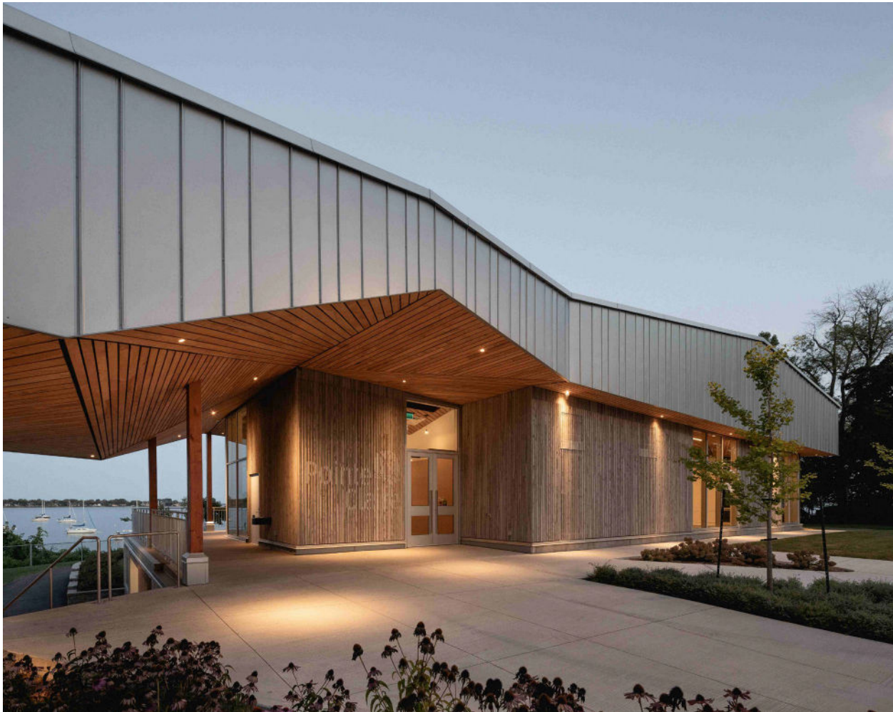
[Photo courtesy of MAC Metal Architectural Inc.]
